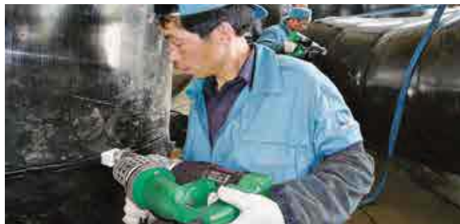
In operation during container construction in China.
